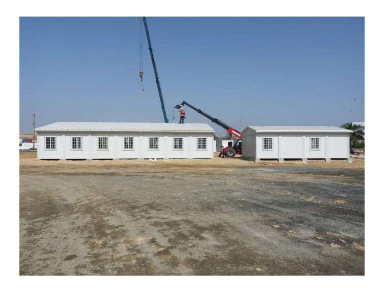
The elements of <u>prefabricated structures</u> (sandwich panels, light steel construction elements, roof elements, stairs and corridors for <u>prefabricated</u> multi-story buildings) have been designed and painted in advance at the **factory** and have been dispatched to the site for mounting. Reinforced concrete flooring is required for
